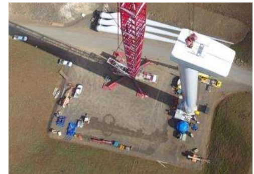
~1,100,000m 2 of hardstands to be constructed
