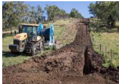
~120km of 33 kV underground cable to be laid
