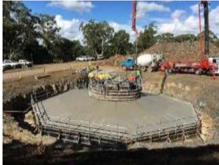
~120,000m 3 of concrete to be poured
