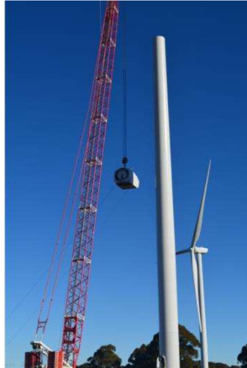
~170,000 tonnes of turbine components to be lifted
